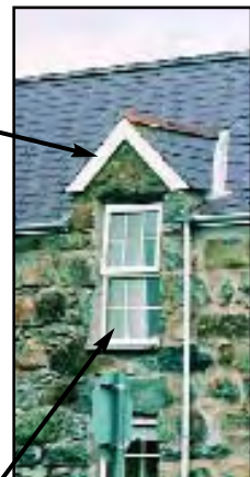
Hard cement pointing, especially of poor quality (left), and ribbon pointing (right), are visually unattractive and can be damaging to stonework: the mortar will crack away from the stones, allowing rainwater and frost to penetrate the wall; it is also non-permeable, preventing the fabric drying out, encouraging moisture penetration through to the inside
