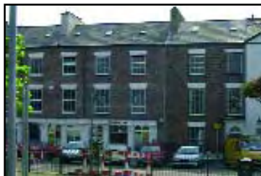
By contrast this new building, which completes an eighteenth century terrace, has shopfronts that replicate the plot widths, are traditional in feel, but are not pastiche; corporate identity is in evidence, but being low key, does not dominate
