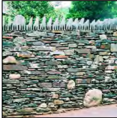
Good use of local materials, good quality detailing and workmanship, ensure that this churchyard wall is appropriate to its location
