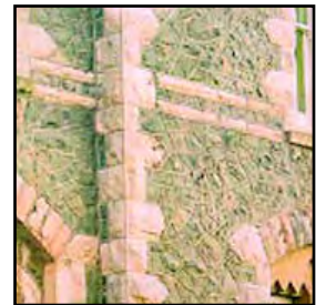
Hard cement pointing, especially of poor quality (left), and ribbon pointing (right), are visually unattractive and can be damaging to stonework: the mortar will crack away from the stones, allowing rainwater and frost to penetrate the wall; it is also non-permeable, preventing the fabric drying out, encouraging moisture penetration through to the inside
