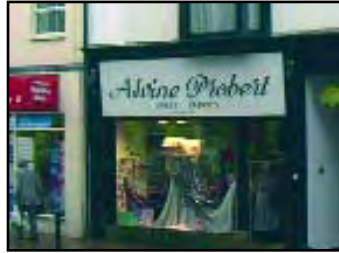
Over-large signs can unbalance a similarly traditional shopfront – high street chains and franchises often promote corporate identity this way
