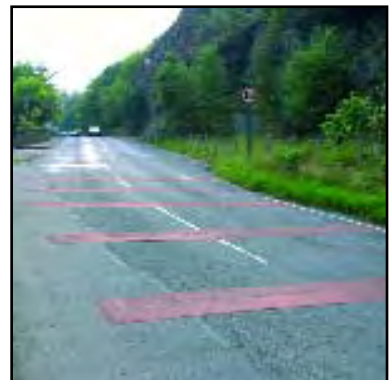
Simple rumble strips at the entrance to villages provide both a visual and aural reminder to reduce speed without being too obtrusive or unsightly
