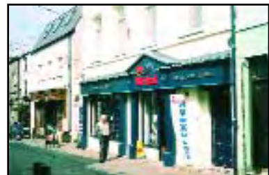
Good modern detailing along traditional lines respects but does not imitate; tidy forecourts and buildings with lively displays make for a welcoming and vibrant commercial district
