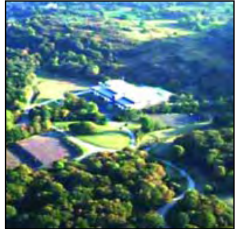
A good example of a development in the countryside which uses the landscape, supplemented by shelter planting, to act as a barrier against visual, noise and nuisance pollution; to modify the climate and aid the energy efficiency of the buildings; to contain and control traffic, and to integrate the built and natural environments
