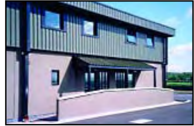
In less vulnerable environments, the use of non-traditional materials may be acceptable, coupled with a high quality specification, and consideration of appropriate colour and weathering characteristics
