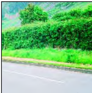
Urban detailing such as standard concrete kerbs should be omitted in favour of a softer margin at verges for country roads
