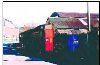
The conversion of small and large scale industrial units can be worthwhile on both sustainable and economical grounds, if suitable uses can be found
