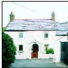
Where an exact replacement may not be desirable, simply styled windows of similar proportion (height to width and glass to frame) are most appropriate
