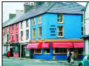
Dutch blinds are always visible even when folded up; they are much more obtrusive than traditional blinds, and do not have the right feel for an established town centre
