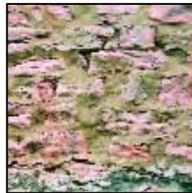
Hard cement pointing, especially of poor quality (left), and ribbon pointing (right), are visually unattractive and can be damaging to stonework: the mortar will crack away from the stones, allowing rainwater and frost to penetrate the wall; it is also non-permeable, preventing the fabric drying out, encouraging moisture penetration through to the inside
