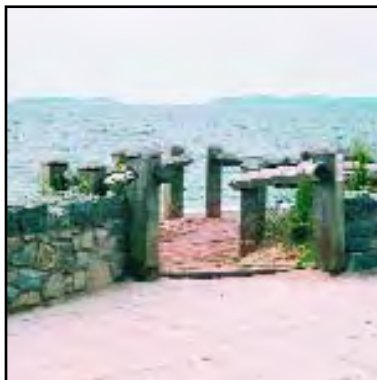
Good street furniture will enhance character - the chunky design of these bollards and railings, the natural stone walling, and the soft surface finish to the path, are a perfect choice for the shoreline
