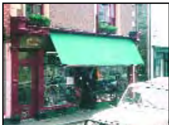
Canvas awnings shield the window contents from direct sunlight but can be retracted fully out of sight into the shopfront when not required
