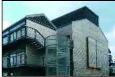
Modern design using materials that respond well to the locality in scale, form, proportion and colour, can produce a very sustainable and ecologically sound development solution
