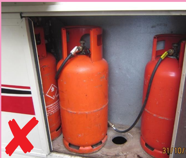
Holes have been made in the bottom of the cylinder compartment for ventilation. The cylinders are also not secure during transit.
