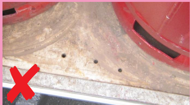
Ventilation holes in the base of the cylinder compartment.
