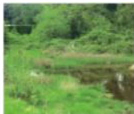
Poorly drained areas
