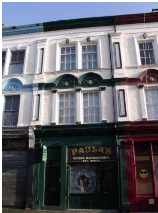
Photo 8: Premises in Bangor Street, Caernarfon
